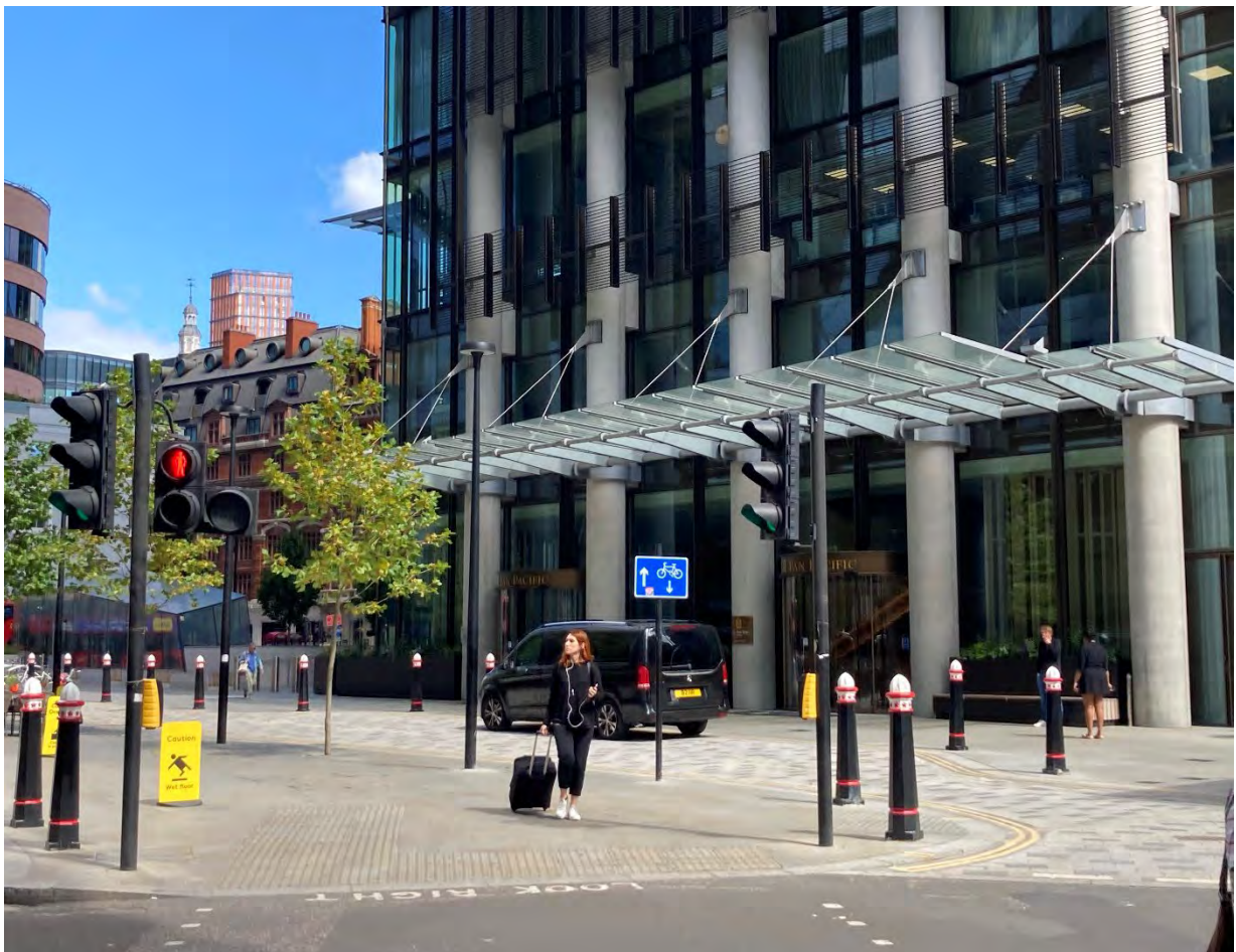
After: The raised carriageway in granite sets on Houndsditch.
