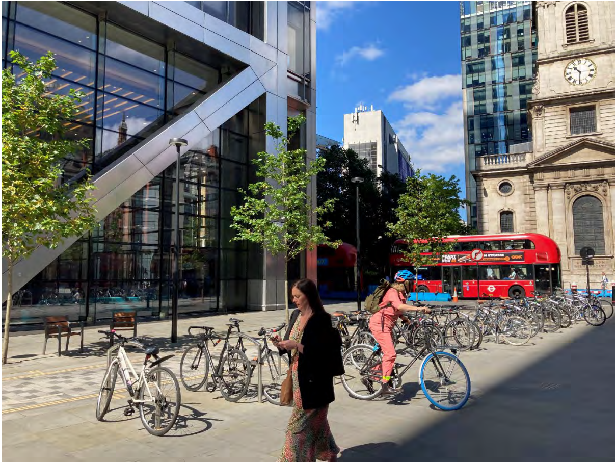
After: The new layout with raised carriageway caters for expected increase in people walking and cycling in the area.
