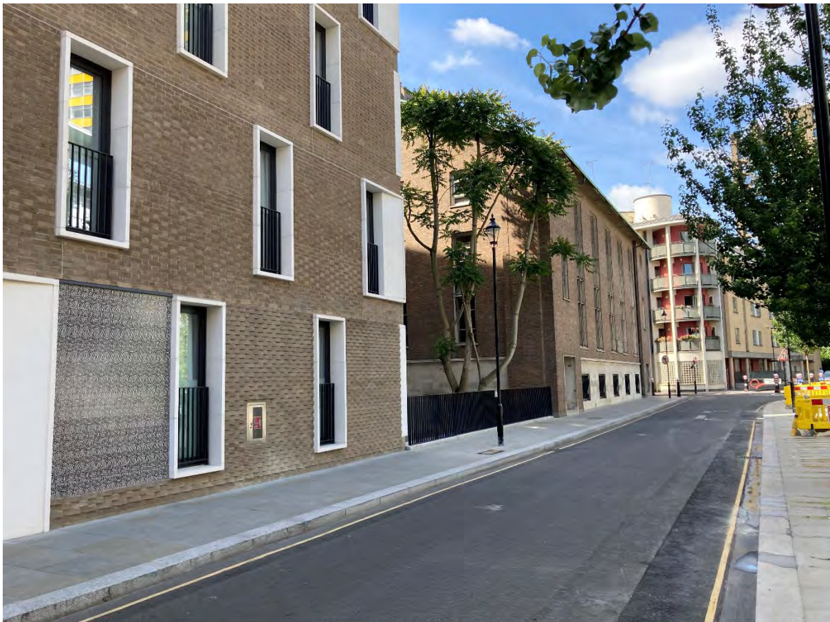
After: Fann Street; the footway adjacent to the development and the church was paved in Yorkstone.
